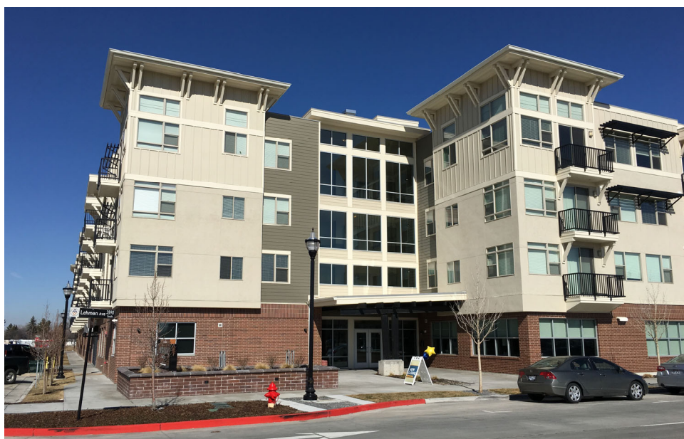
Apartments within the City Center Zone
