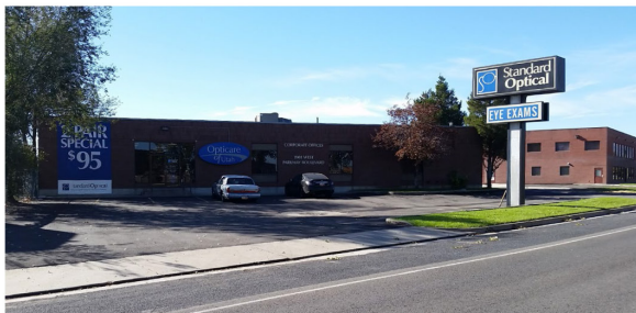
Image 1 Existing Commercial Building
